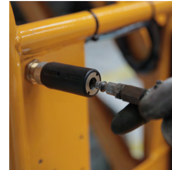
5 Compressed air line
